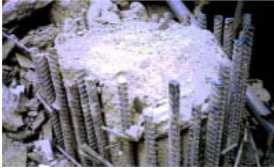
Fig.10 Lap splices failure of rectangular Column
