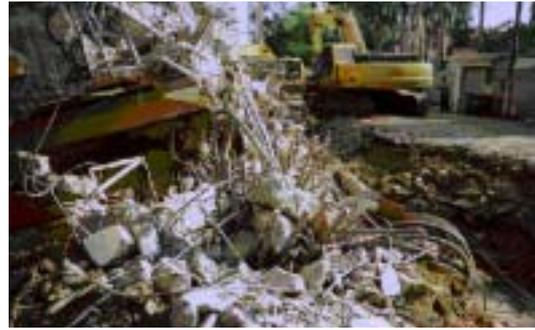
Fig.11 Lap splices failure in a collapsed building
