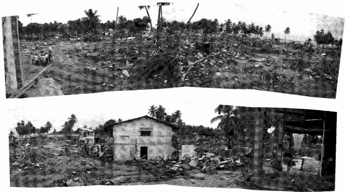
Figure 9. Hambantota: Masonry houses located within a few hundred meters from the coast were completely destroyed, a few more recently constructed houses had less damage.
