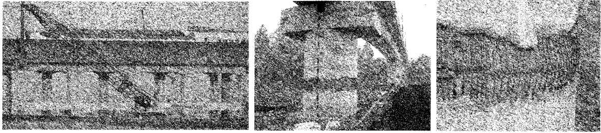
Photos.8-10 Failures of JR-Shin-kan-sen during the 2004 Niigata-Chuetsu earthquake.
