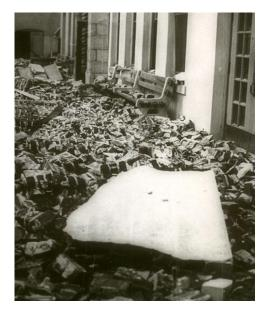
Figure 2 Polytechnic High School: Fallen Brick Debris over Exit Corridor after Long Beach Earthquake, 1933. Safe passage for exiting buildings must be provided during building design.
