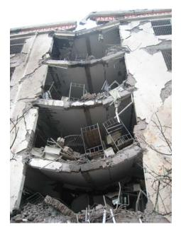
Figure 7 Large deflection of cast-in-situ RC beams and slabs of floors (7/11)
