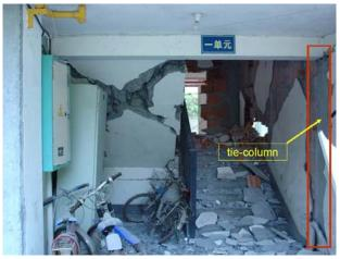
Figure 15 Damaged stair shaft of a residence building of masonry structure in Mianzhu City (7/8~9)
