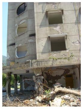
Figure 4 Damaged bottom RC frame structure (7/9)Note: (7/9) = (zoning intensity/estimated intensity)
