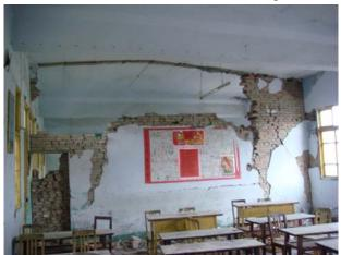
Figure 10 Remaining pre-cast RC floor (7/9)
