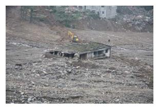
Figure 3 A 4-story apartment building mostly buried by debris flow late Sept.2008 in Beichuan County
