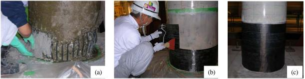
Figure 5 Repair by CFS Jacketing with Quick-Drying Materials: (a) Repaired by MMA Mortar, (b) CFS Jacketing with MMA impregnation resin, and (c) Completion of Repair
