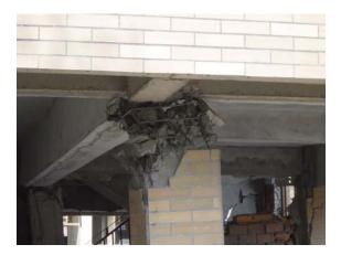
Figure 6 Plastic hinges of a frame structure (7/11)
