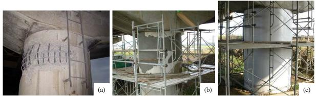
Figure 1 Seismic Damage and Its Repair by Carbon Fiber Sheet Jacketing: (a) Damage, (b) Repaired with Mortal, and (c) Completed with Carbon Fiber Sheet Jacketing (National Institute for Land and Infrastructure Management and Public Works Research Institute, 2006)
