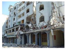
Figure 5 Damaged upper walls of masonry building with bottom RC frame structure (7/9)
