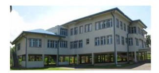
Fig. 1. A tsunami resistant building with elevated lower level in Sri Lanka.
