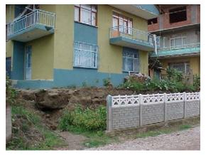
Figure 7 Lack of Secondary Ground Deformation on the Footwall of the Normal Fault Movement near Golcuk during the 1999 Kocaeli Earthquake
