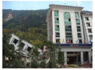
Figure 13 Sequence collapse caused by collision between office and apartment buildings in Beichuan County (7/11)
