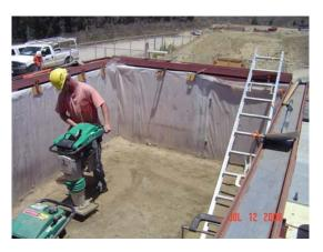
Figure 4: Backfilling and compaction inside soil container
