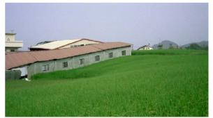
Figure 6 Ground Warping Associated with the 1999 Chi-Chi Earthquake (photo by N. Sitar)
