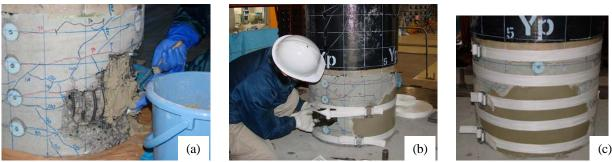
Figure 6 Repair by Fiber Band Jacketing with Mechanical Anchors: (a) Repaired by Mortar, (b) Tightening Bands with Mechanical Anchor, and (c) Completion of Repair
