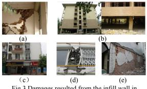
Fig.3 Damages resulted from the infill wall in Wenchuan Earthquake
