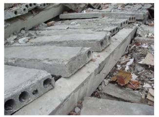
Figure 9 Fallen RC beam and pre-cast floor slabs (7/9)
